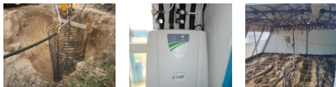
Fig.2 The components of the heating system of the third insulated greenhouse: (a): the Conic Basket Geothermal Heat Exchanger (CBGHE), (b): The geothermal heat pump (GHP), (c): a multilayer heat exchanger system.
